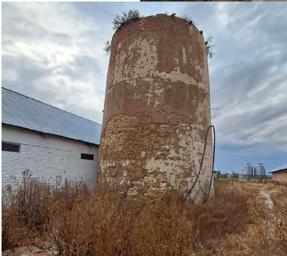
Figure 14&15: Worker's house in back - granary behind the historic section of the first barn
